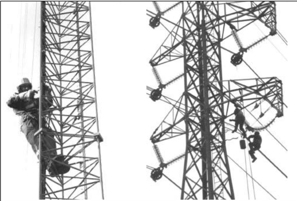
*Figure 8. Electricians working on the maintenance of telecommunication mast (left) and on the assembly of an electricity transmission mast (right).*
